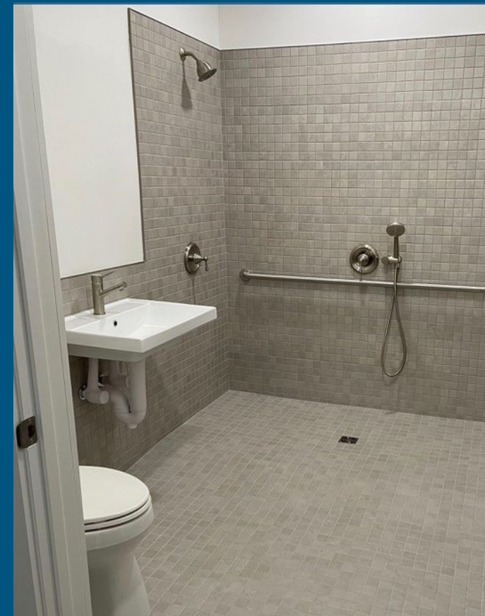
ADA Accessible Bathroom with Shower
